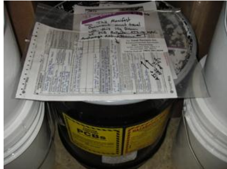
DOT approved shipping manifests and haz-mat container of PCB ballasts ready for shipment
