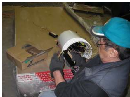
Village maintenance staff double checking ballasts for PCBs
