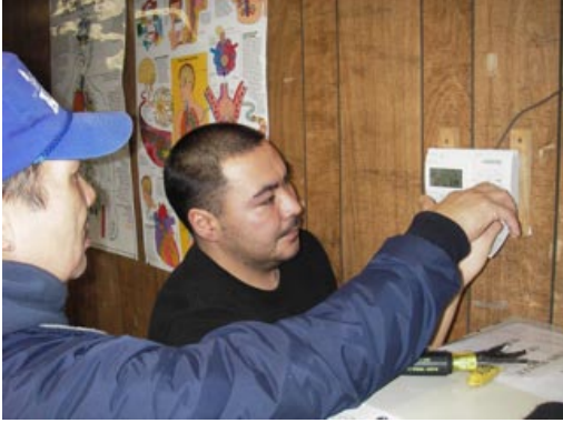
Maintenance staff installing and programming new thermostats
