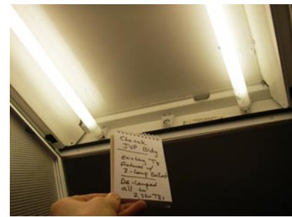
Energy use was reduced by 31% by simply removing one existing T8 lamp from each fixture
