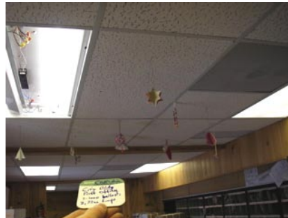
2-lamp electronic ballasts and 32-watt T8 lamps
