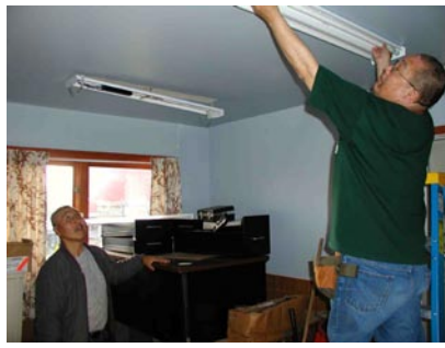
Clifford Whitman and Alvin David work on a light fixture.
