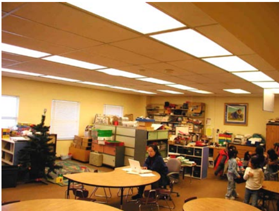
Classroom T8s in classroom.
