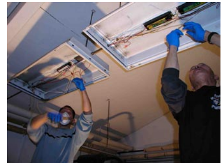
Wilson Tikiun and Jerry Chris upgrade light fixtures.
