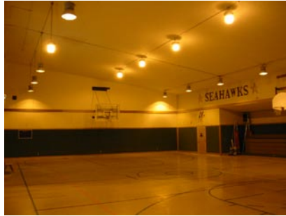
Existing 157 watt HPS lighting
