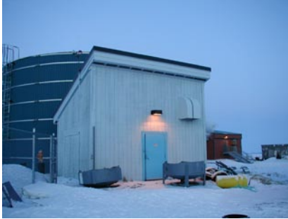
Golovin – BSSD water plant
